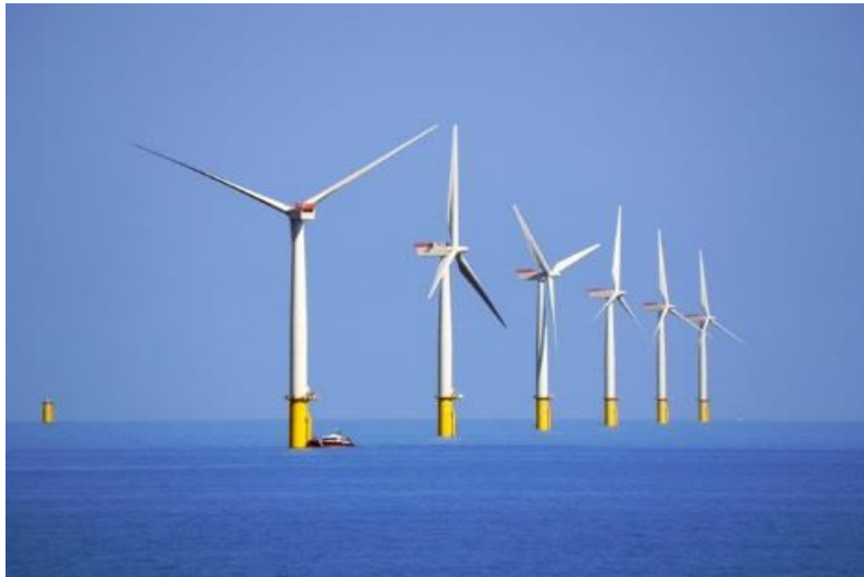
Walney offshore wind farm, UK
